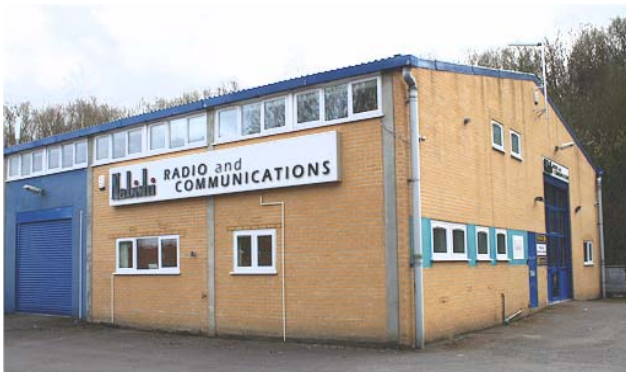
Headquarters in Reading
